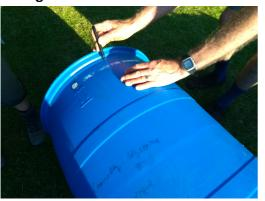
Empty residue from the barrel into buckets and spread out tarpaulin to catch the bits of plastic, rinsing if necessary. Next drill a hole for the down pipe to fit into the barrel lid – make sure to locate the hole so that your pipe will go in without any angle problems.
