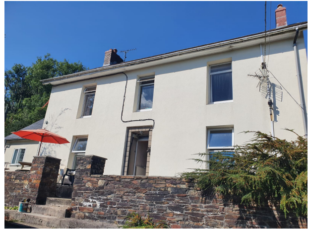
The farmhouse at Maesgwyn Isaf (Image credit: Ecological Land Cooperative)
