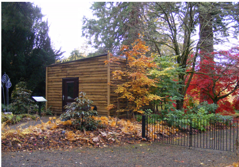
Above and below: Turbine house at Dawyck Garden
